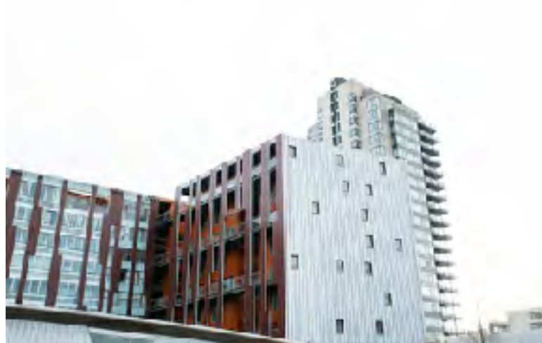
Smart retrofitting for Urban Housing
